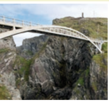
Mizen Head Bridge
