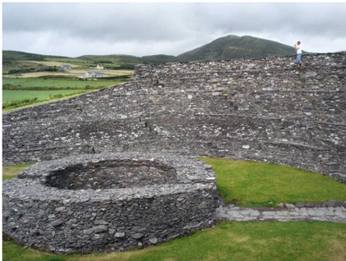
The 2,000-year-old walls of Ireland's Leacanabuaile Ring Fort have withstood the test of time – without the aid of mortar or cement. PHOTO BY RICK STEVES
